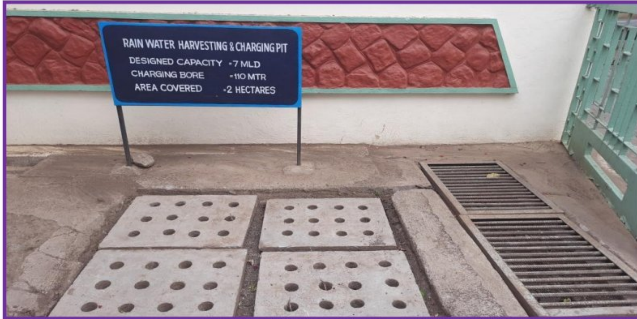
Sample Name Board in front a Rain Water Harvesting System
